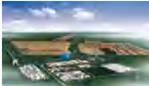
Zhundong Coal Power Energy Base (Xinjiang)
