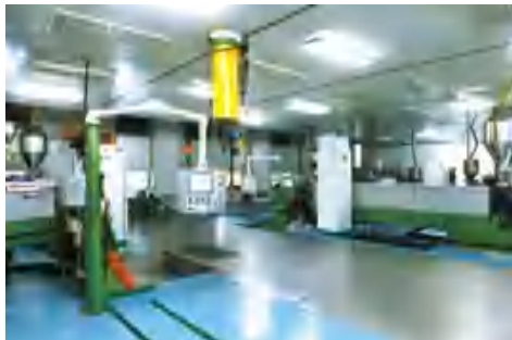
500kV VCV Production Line From Switzerland
