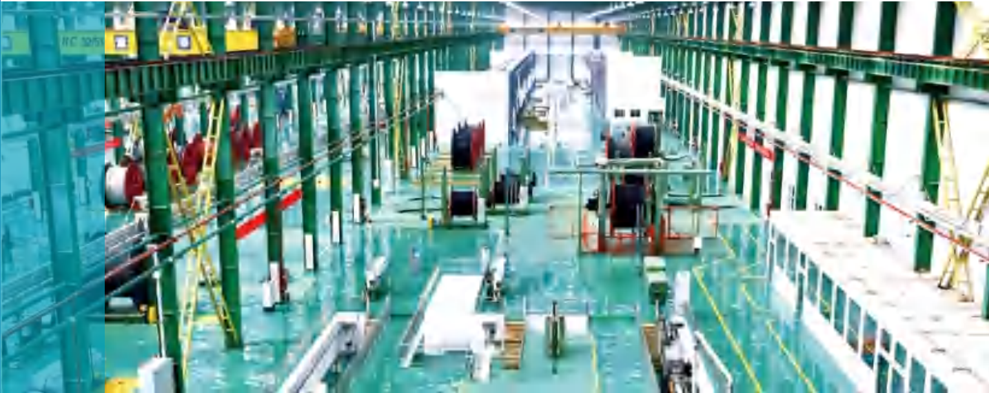
Panorama of HV Cables Workshop
