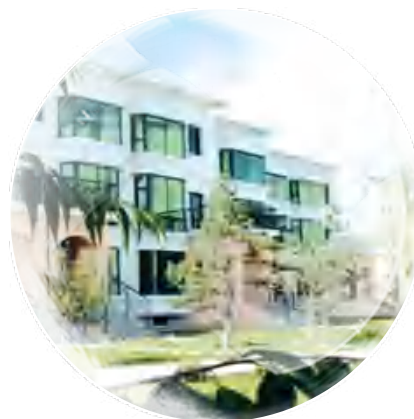
Solar Central Heating and Enlightening Systems for National Comfortable Housing Demonstration Project
