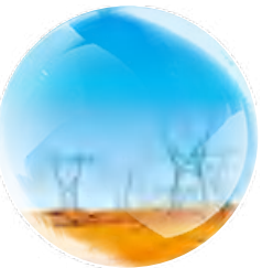
Package Project of 110kV - 220kV Power Transmission & Transformation Line in Sudan
