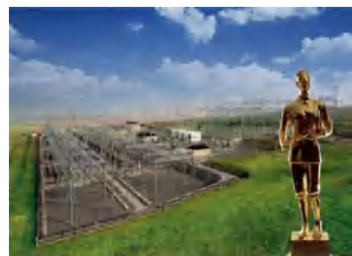
500kV Substation in Khudzhand Tajikistan
