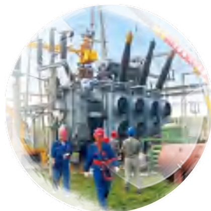
Emergency Maintenance for Electric Line at Disaster Site
