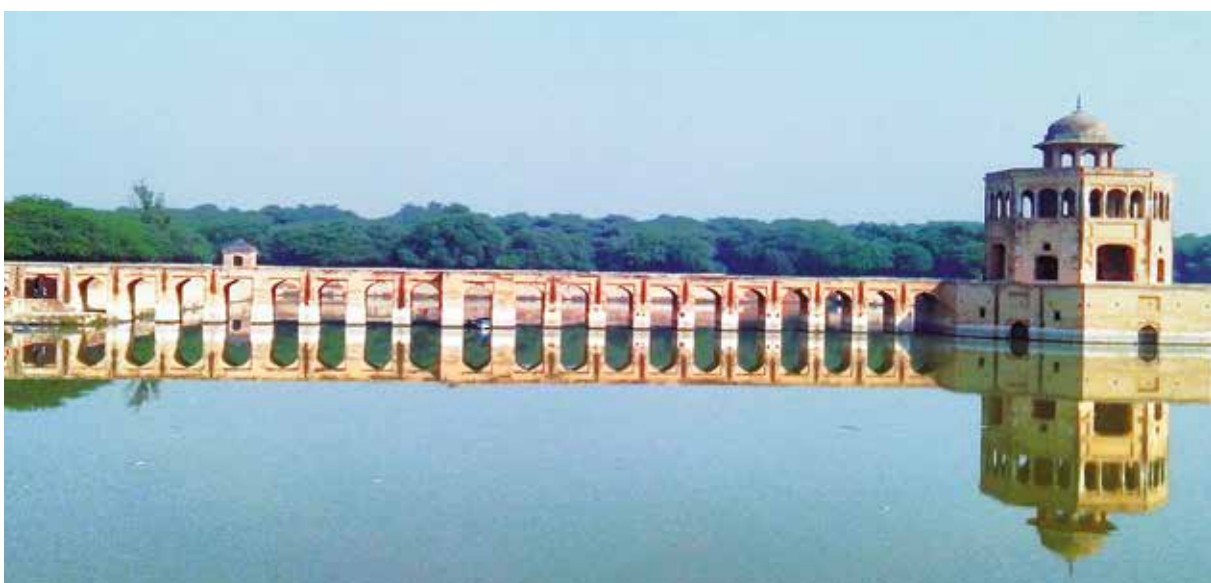
Hiran Minar Water Tank, Sheikhupura
