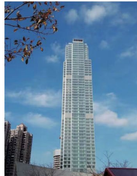
Street no. 60, jing an district, Shanghai quantity: 38000 m 2 Glass Makeup: Triple Silver Low-E laminated insulating glass
