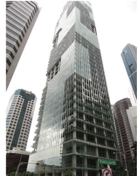
Market Street, Singapore Quantity: 20000 m 2 Glass Makeup: Triple Silver Low-E laminated insulating glass
