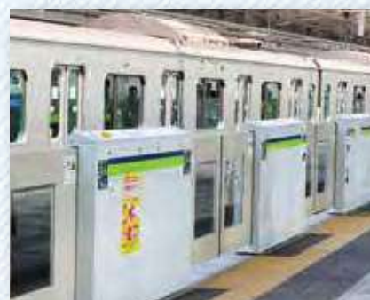
Automatic platform gates
