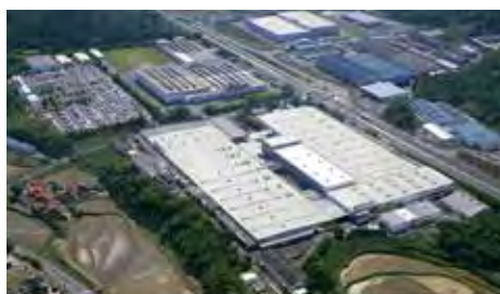
● Yamaguchi Plant 山口工場 Site: 187,182 m 2 (2,014,810 sq.ft.) / Floor space: 68,515 m 2 (737,490 sq.ft.)
