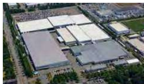
● Yamagata Plant 山形工場 Site: 175,294 m 2 (1,886,850 sq.ft.) / Floor space: 103,665 m 2 (1,115,841 sq.ft.)
