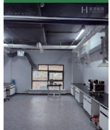
Electrolyzer R&D and Testing Center
