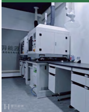
Membrane electrode assembly R&D and Testing Center
