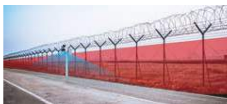
Airports Perimeter Security
